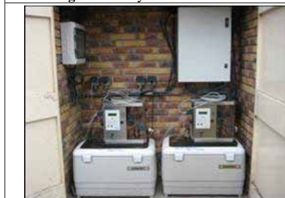
Figure 5. Two automatic samplers Bühler 1029
